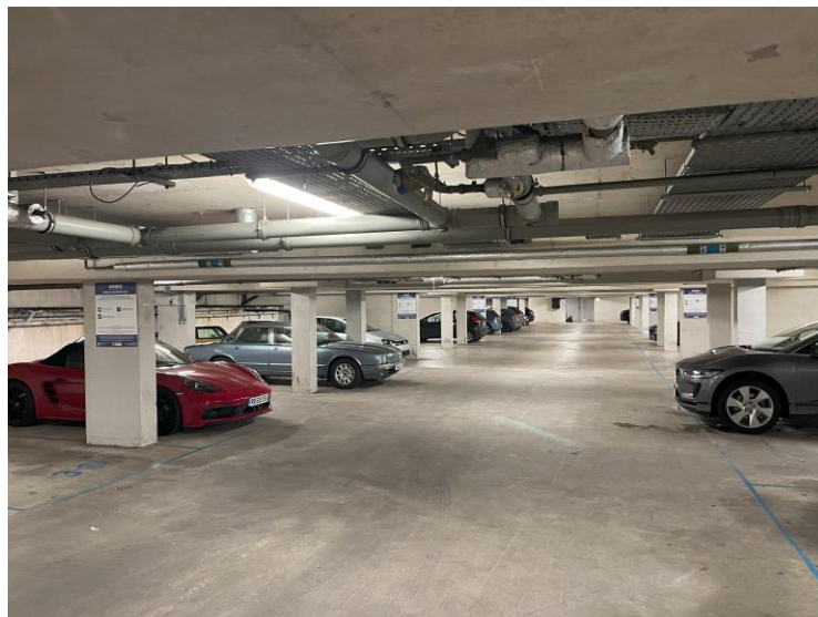
8) Example of basement car park
