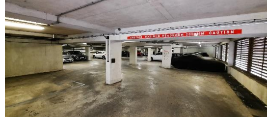
Figure 4 - Typical car park view.
