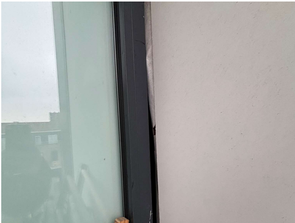
Photograph 22 - Gap Between External Finishes Level 6 Gridline 7D
